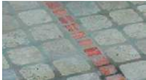
AGED MARBLE FLOORING BEFORE THE FINAL CLEANING POST-INSTALLATION
