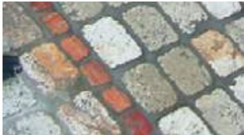
SURFACE AFTER THE FINAL CLEANING POST-INSTALLATION WITH DETERDEK
